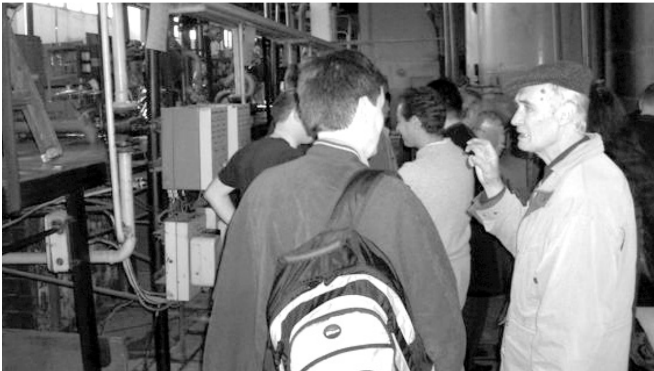
Boiler house in Almaty district heating system.
