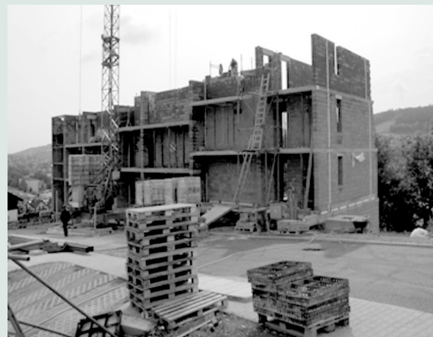
Efficient House under construction in Susice
