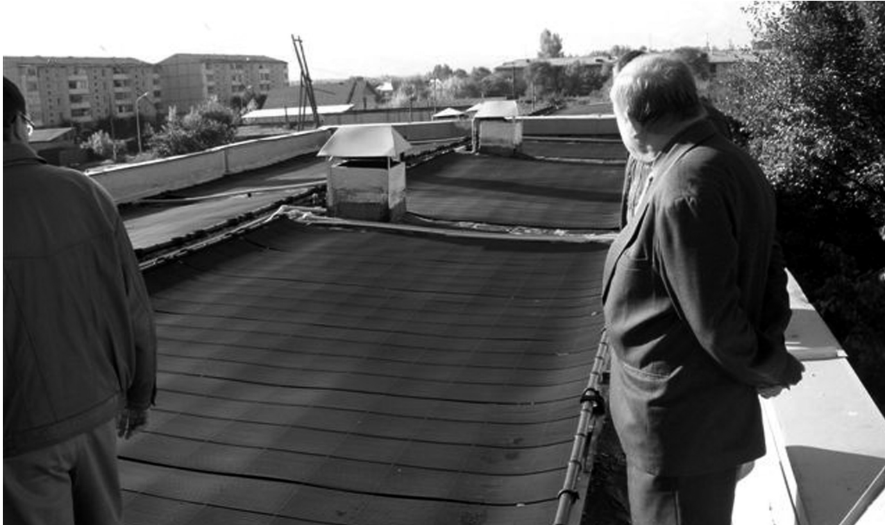
District heating system with a solar preheater on the roof ( Almaty).
